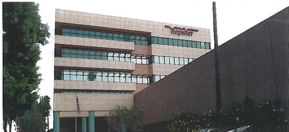
Register building: Freedom Communications sold 173,000-square-foot headquarters for $27 million with lease-back
